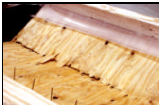
Left: (a) roof sheathing nailing test using a vacuum
