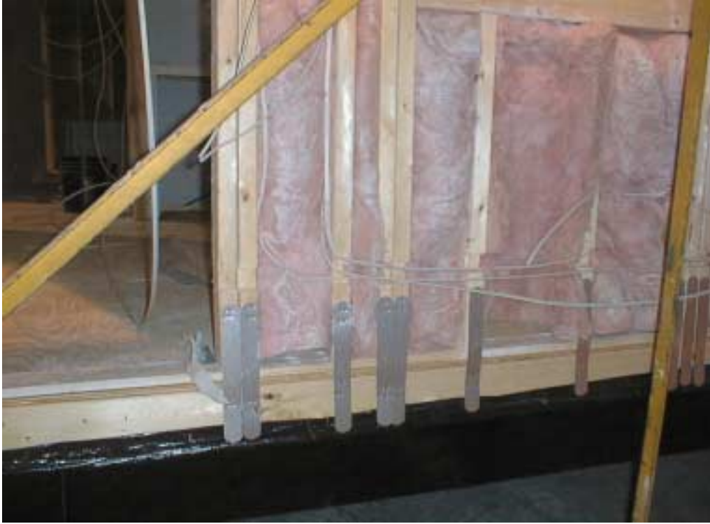
20 gauge ties securing studs to floor frame.
