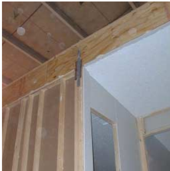
Strap-tie connecting interior wall to primary structural beam.
