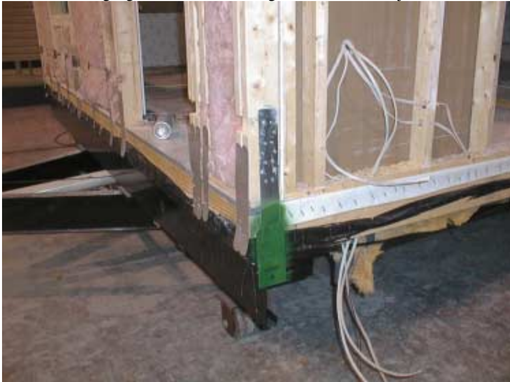
Shear wall strap connector on interior wall of home.
