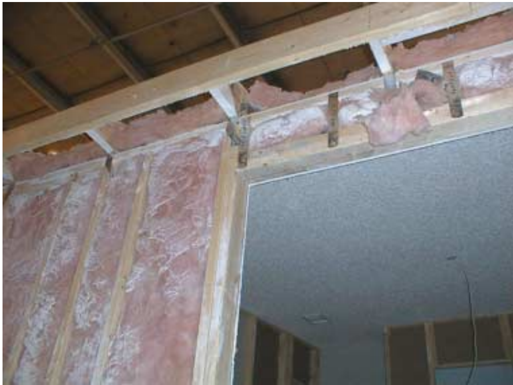
20 gauge ties securing studs to floor frame.
