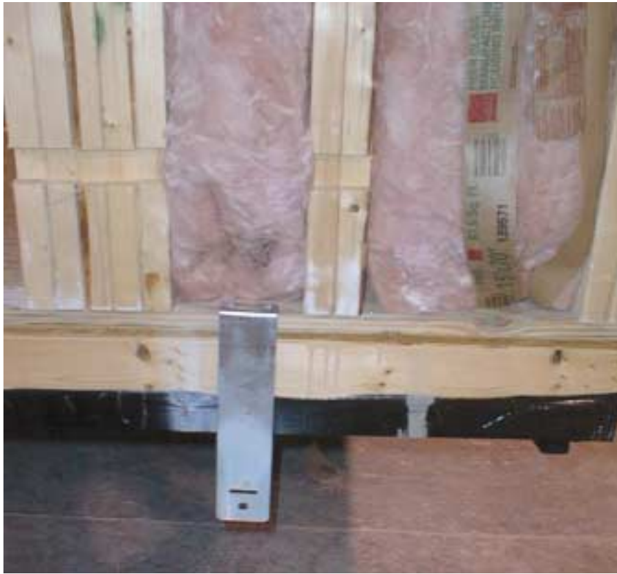
Tie-down connector attached to floor framing.
