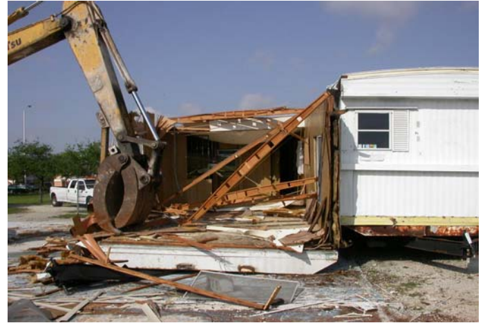
Figure 3. Backhoe demolishes one mobile home
