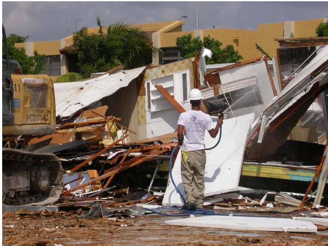
Figure 4 Wet demolition is in process using mist-controlling nozzle
