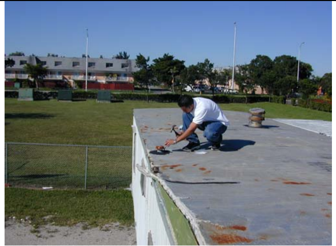
Figure 2. Inspector collecting samples on the roof of one mobile home for asbestos analysis
