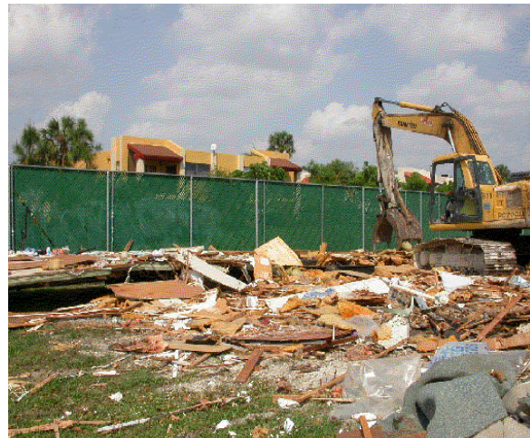
Figure 17. HCET test facility after complete demolition of mobile home units.
