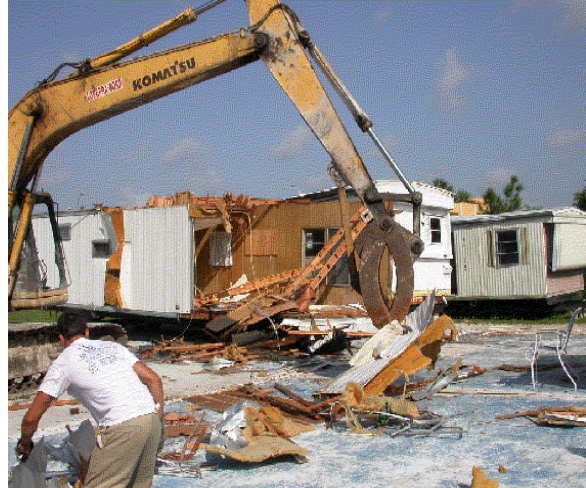
Figure 11. Backhoe segregating the wood from a mobile home unit.
