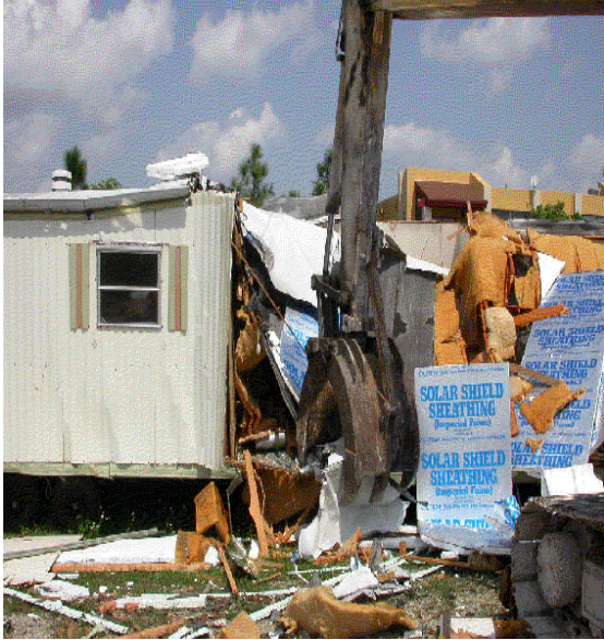
Figure 14. Backhoe separating the insulation materials.
