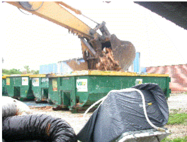
Figure 21. Dumpster collecting wood debris.
