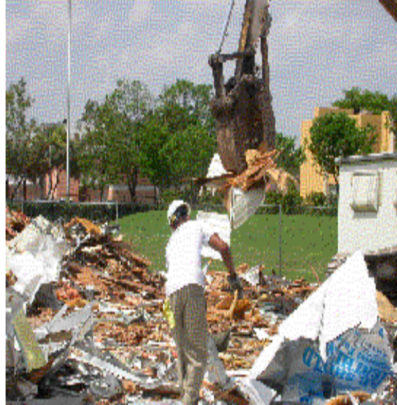
Figure 15. Backhoe crushing the outer walls of a mobile home unit.
