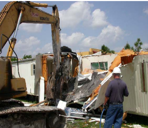
Figure 12. Wet demolition of a mobile home in process.
