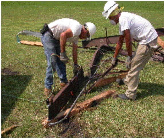
Figure 16. Steel axles were broken into pieces using torches.
