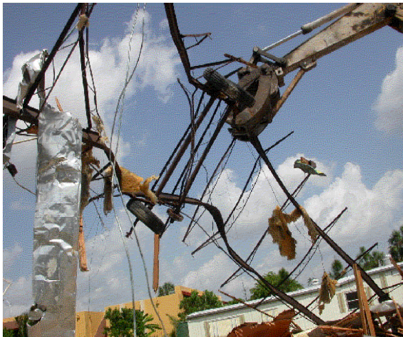
Figure 13. Backhoe lifting the steel axles and frames.
