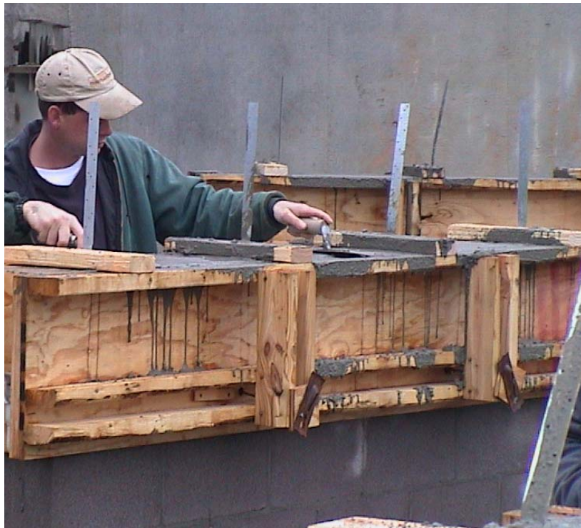
Figure 7. Simpson Strong-Tie HETAL 20 Placement in Reinforced Concrete Tie Beam.
