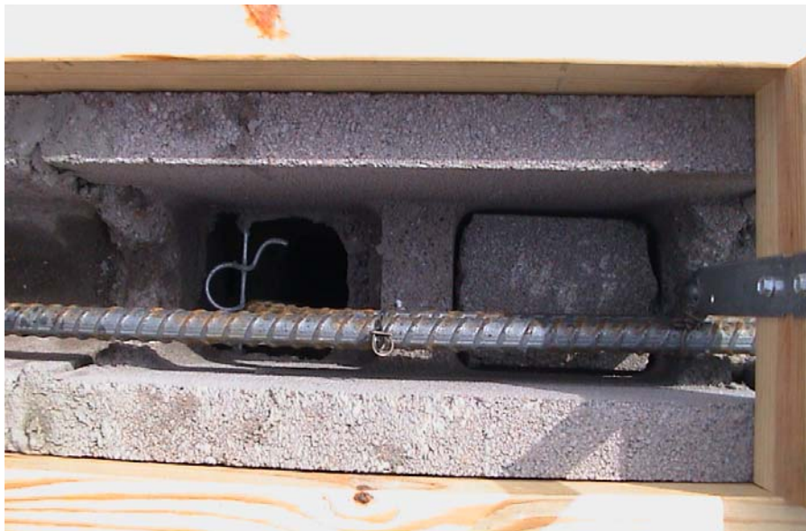
Figure 5. Reinforcing Bars in Top of CMU Bond Beam.
