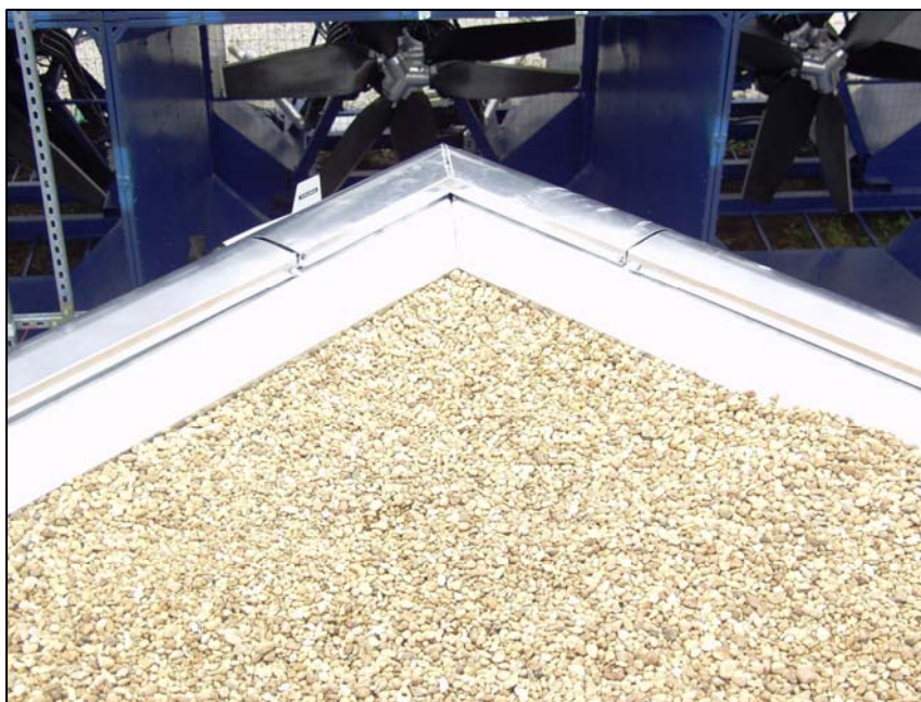
Figure 34. Gravel Scour Associated with FRAC1 AeroEdge™ Shape at 3000 rpm
