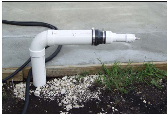
Figure 8. Three in PVC Pipe Extended from Reference Pressure Line
