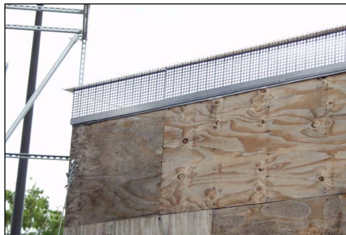
Figure 25. Test Structure Equipped with Flat Roof AeroEdge Guard
