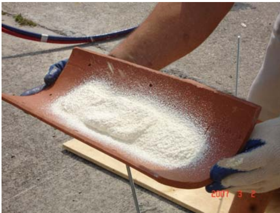
Figure 3.2: Typical Foam Installation
