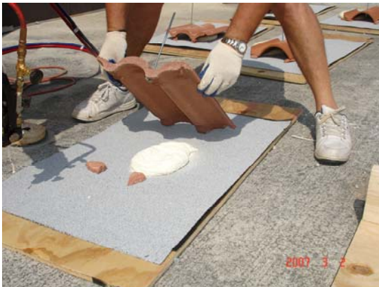
Figure 3.13: Deck Underlayment System
