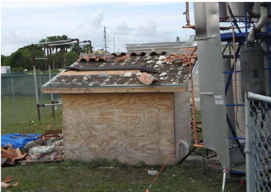
(b) Roof Conditions Subjected to 120 mph Wind Speed at 50^{\circ} Direction
