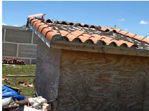
(b) Roof Conditions Subjected to 120 mph Wind Speed at 50° Direction
