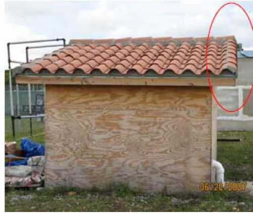
(b) Model 1b: Clay Tile Roof with Foam and Extra Side Ridge Tiles
