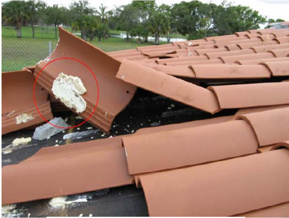
(a) Clay Tile Roof with Foam in Model 1a
