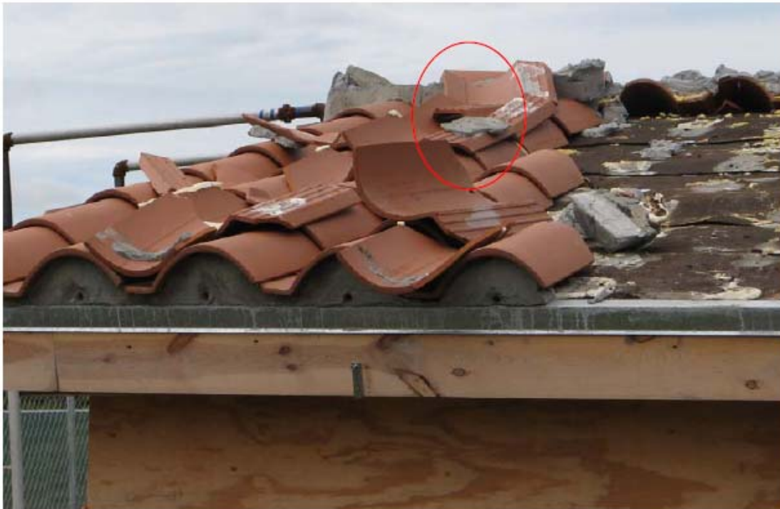
(b) Clay Tile Roof with Mortar in Model 2
