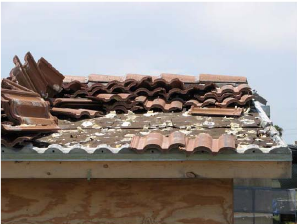
(b) Roof Conditions Subjected to 120 mph Wind Speed at 50^{\circ} Direction
