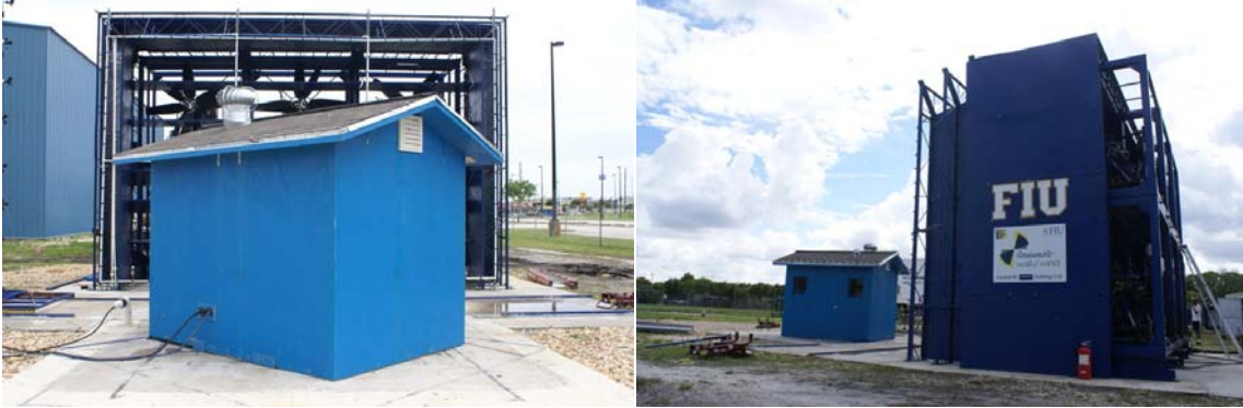
Figure 1: Low-rise building with gable roof in front of WoW in a testing position
