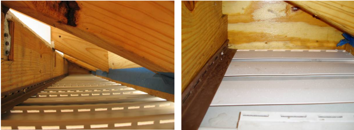
Figure 11 Hidden Vent Soffit (original on left) with the deflectors (modified on right)
