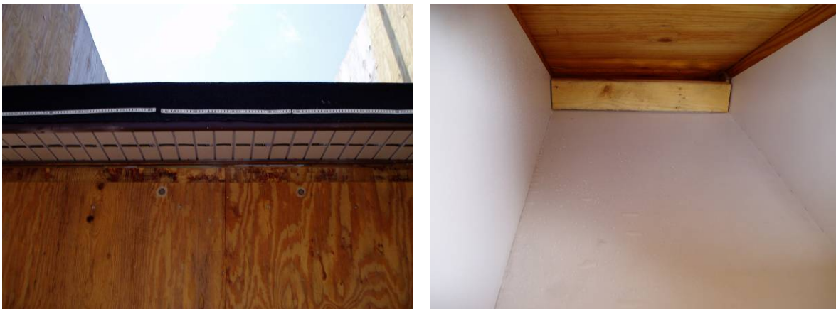
Figure 12 Slot Vent and Baffle System (Existing Soffit Vents were Sealed)
