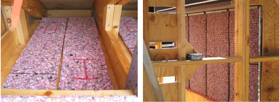
Figures 13 A Poor Choice for Wetting Measurements: Carpet Rebond
