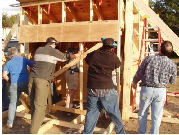
Figure 4 Installation of Soffit Rig
