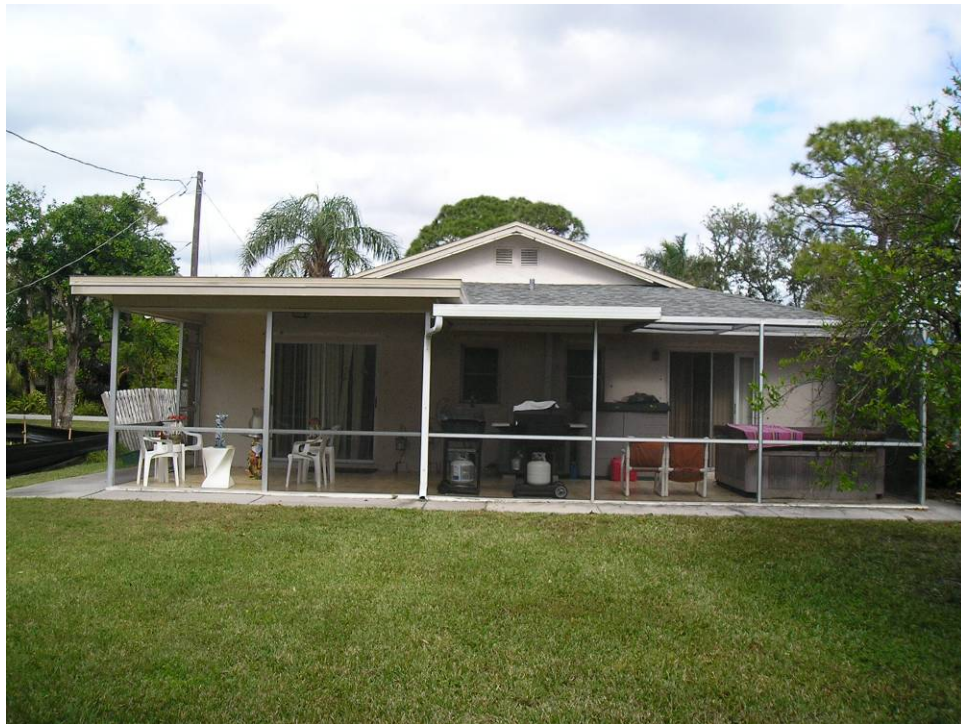
Figure 11. View of Prototype FL-19 Attached Porch at Rear of House.
